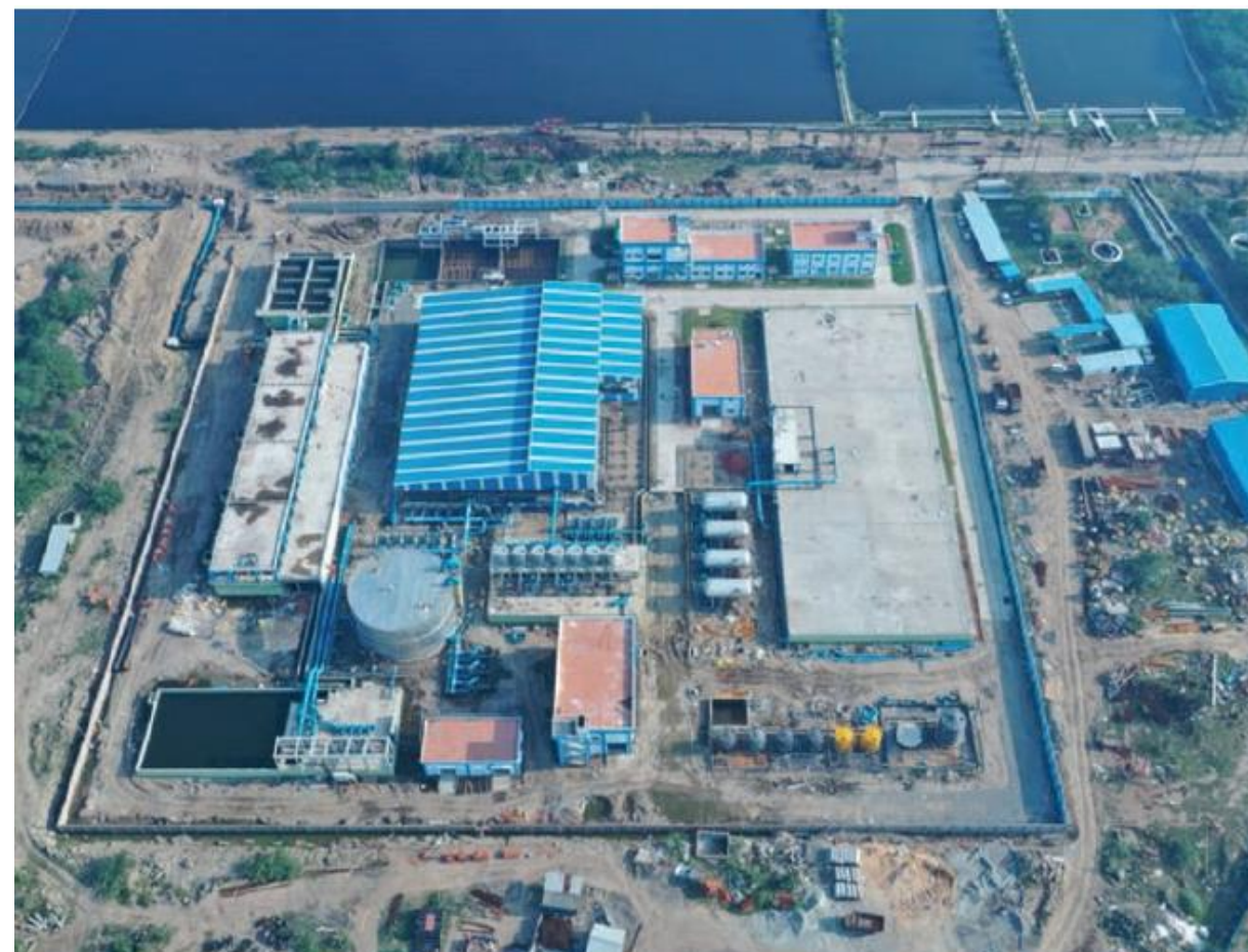
Tertiary treatment plant at Kodungaiyur (CMWSSB)
